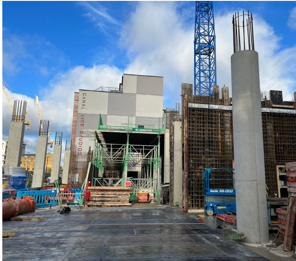
Construction underway at LBIC's state-of-the-art Apex facility
