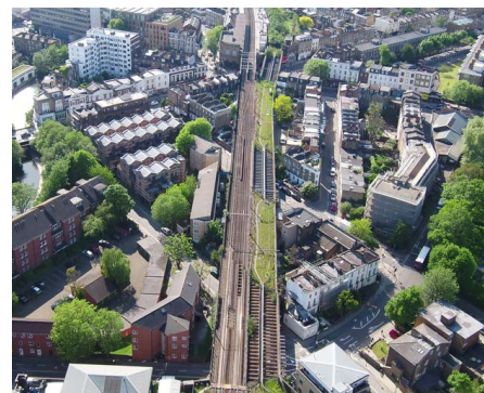
An aerial view of the Camden Highline
